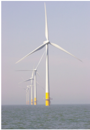
Offshore wind turbines. Pretty? or not?
